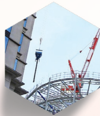
New Build Construction
