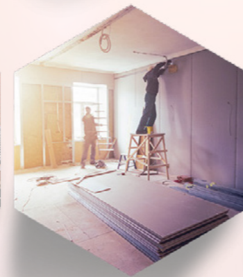
Refurbishment & Fit Out
