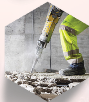
Strip Out & Demolition
